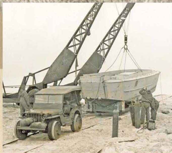
Above: Jeep with flanged wheels on the 58-inch gage track was used to pull the landing craft on the rails from the beach.
