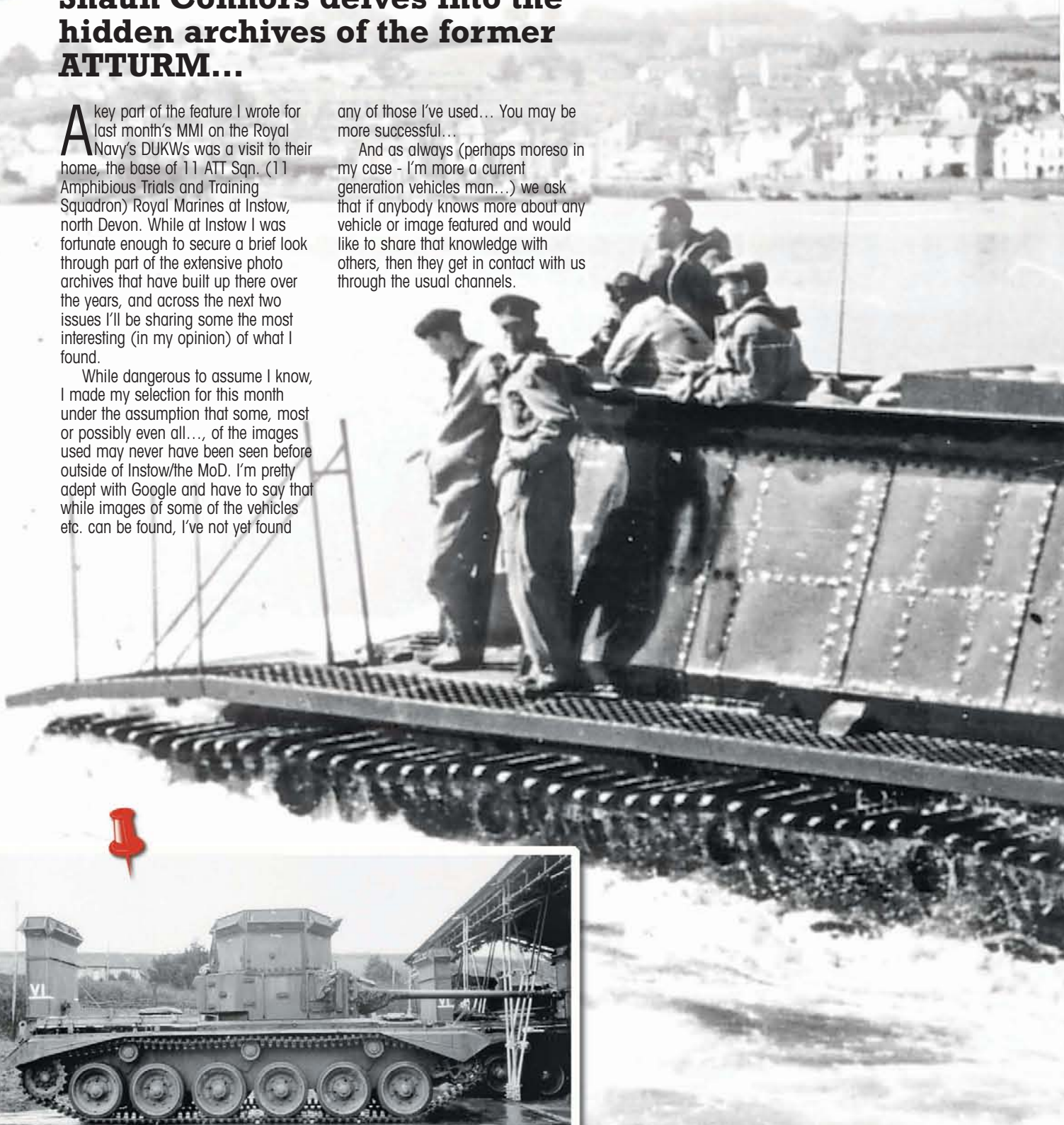
Left: the A34 Comet was probably the best British all-round tank to see service during WW2 and the type remained in service with the British Army until 1960. Shown in this undated image is a Comet fitted with what appears to be a semi-permanent wading/fording kit.
