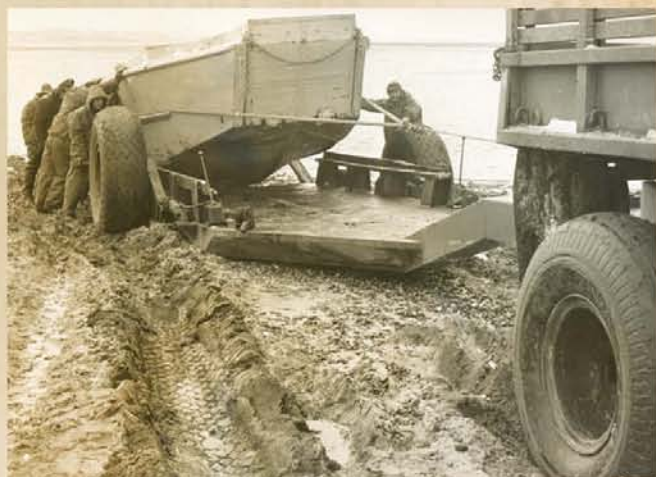
Above: around December 1942, the LaPlante-Choate retractable wheel pole-type trailer is seen here being loaded with the landing craft for the test.
