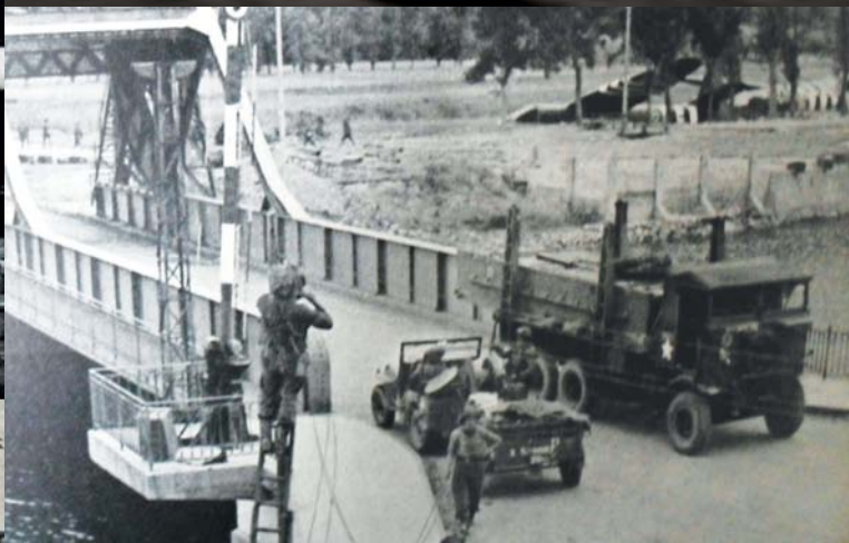
This Terrific shot shows a Retriever Recovery Wagon in 1942, note the extending gantry above the driver's head.
